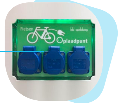
Powerplugs for charging electric bikes (optional)
